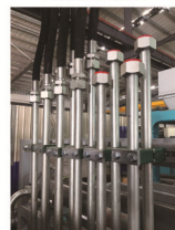
Non-Welded Hydraulic Hose Connections 非焊接液压管路
